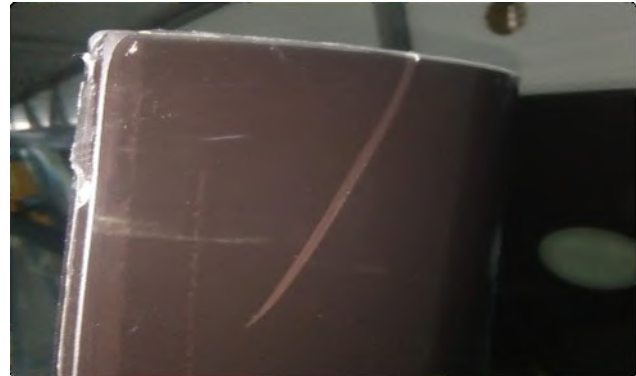
Fig. 5 – A crack resulting from the deviation in geometry of the inner glass layer after the autoclave
